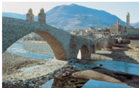
Hump-back bridge over the river Trebbia, 9 th cent., Bobbio
